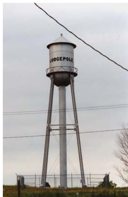
Lodgepole water tower, 2001 Photo.
