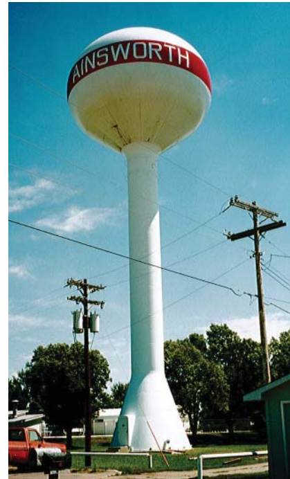
Ainsworth water tower; 2001 Photo.
