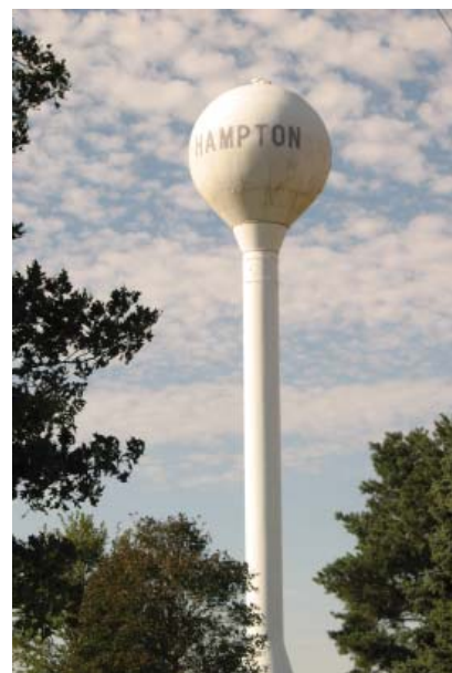
Hampton water tower, 2010 photo.
